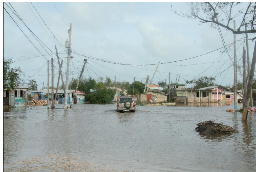
Figure 1. Hellshire Fishing Village, Portmore, Jamaica. One day after the passage of Hurricane Dean (August 2007)
