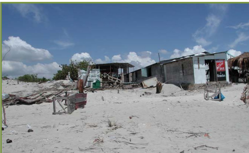
PLATE 3 Destruction of wooden structures at (built approximately 30 – 40m from the shore) along the Hellshire beach.
