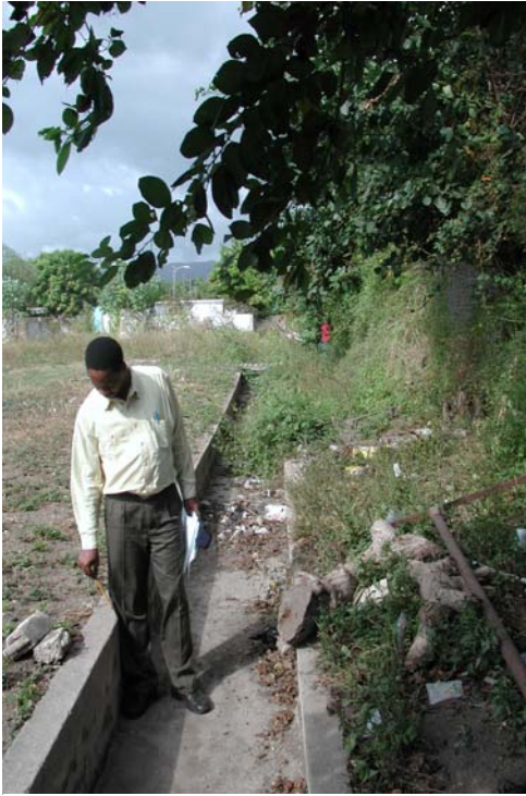
Plate 9: Showing poor maintenance of drains with in Caymanas Gardens D Scale: 175 cm
