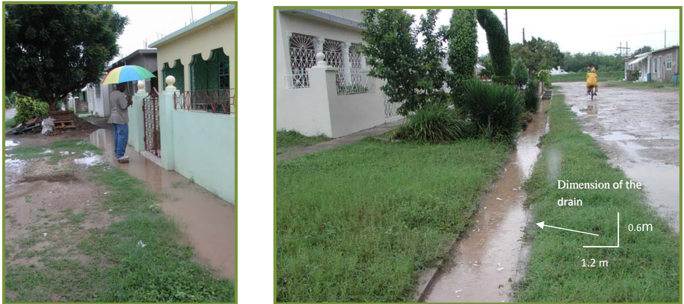
PLATE 13: The Flooding Potential of Christian Gardens. This shows the amount of water settling and rising after thirty minutes of rainfall. The dimension of the drains is 0.61 m in depth by width of 1.2 m. There is a high potential for flooding with Christian Gardens
