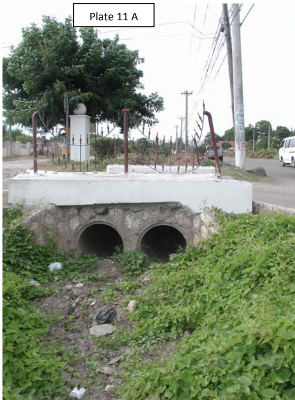
Plate 11 A& B: Showing poorly maintained drains along Gregory Park Main Road
