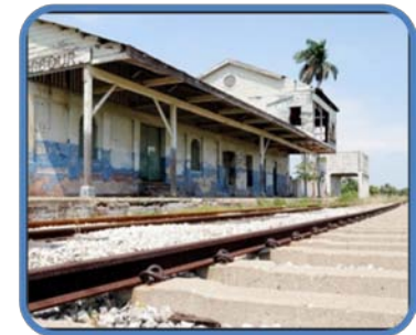
Old Harbour Railway Station
