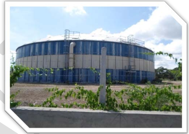
Figure 19: NIC Water Storage Tank by Jobs Lane Spanish Town
