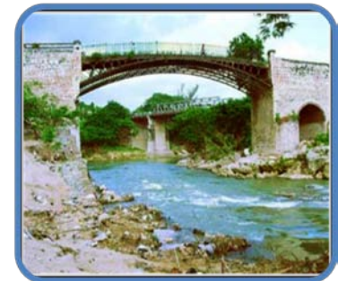
Cast Iron Bridge
