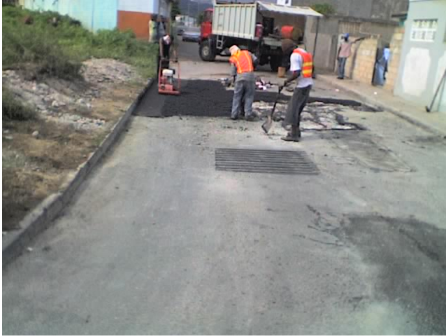
In-house Road Patching Exercise – Top of Germaine Rd.
