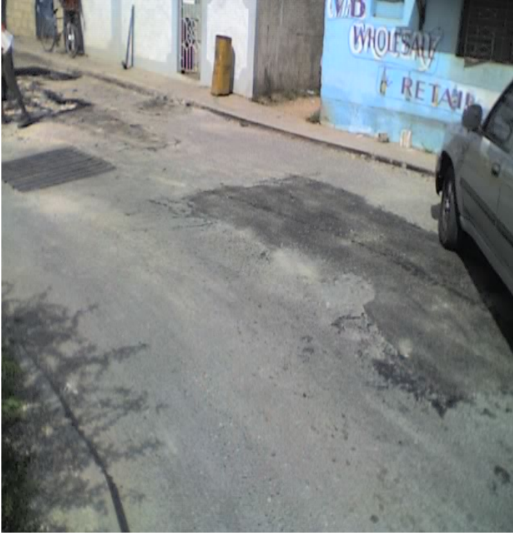
In-house Road Patching Exercise
